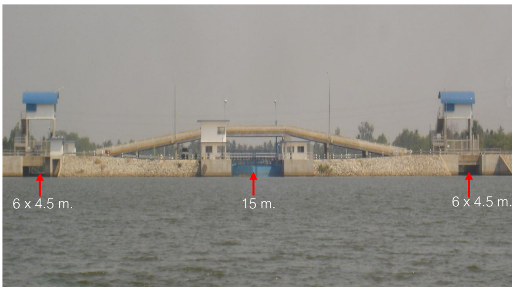
Figure 2 Closure Dam Gate
